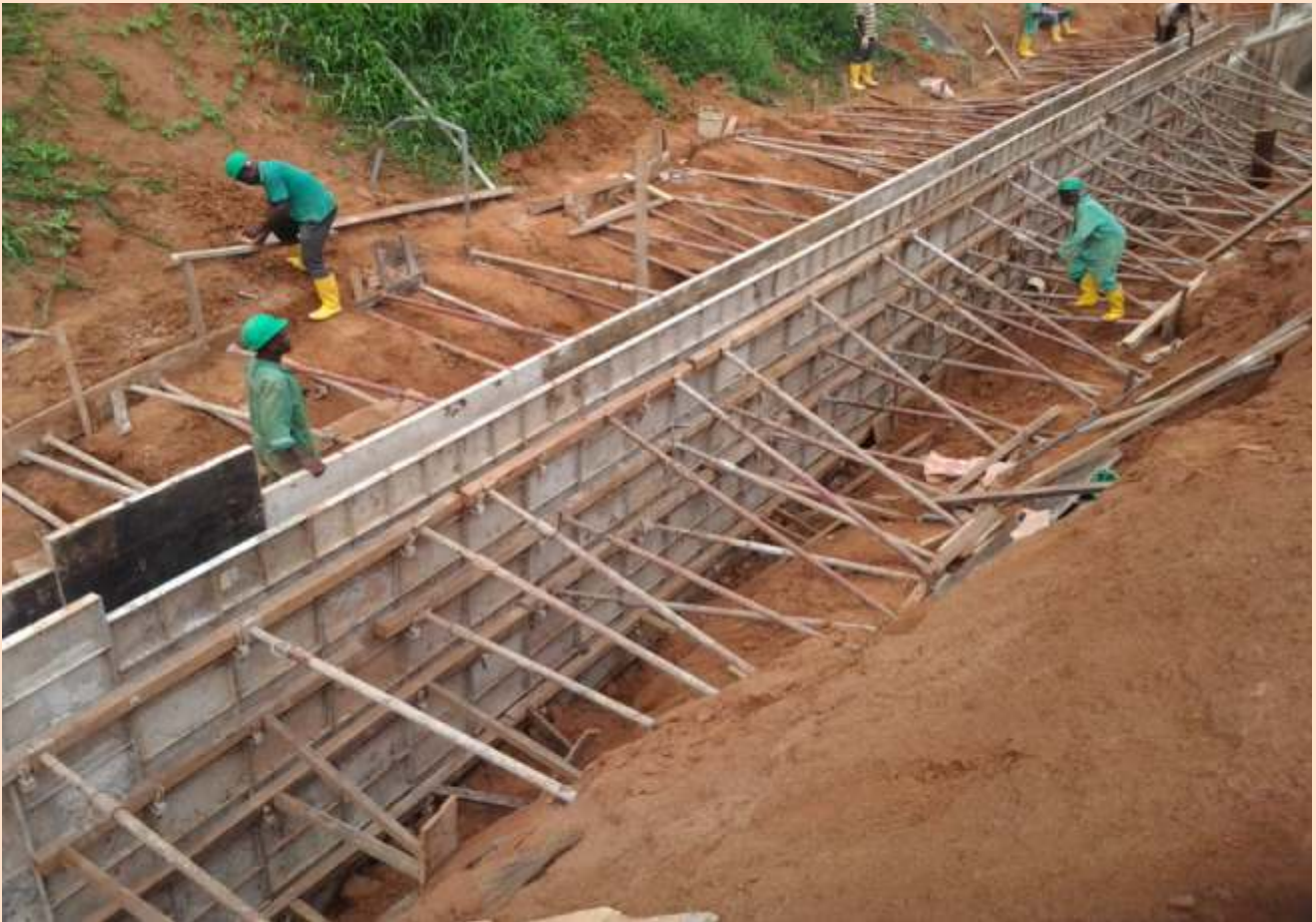
Retaining Wall Construction For Asphalt Road At Height Different
