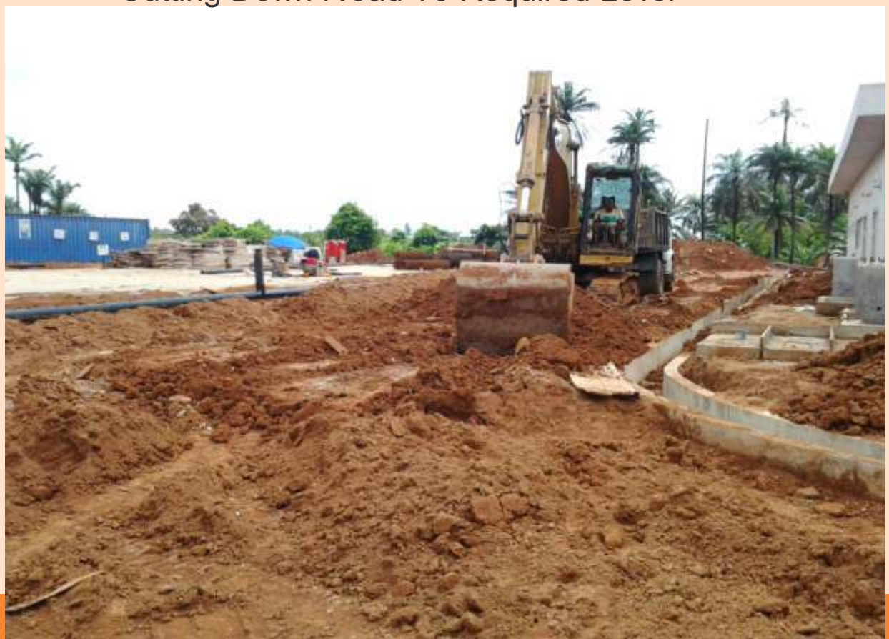
Cutting Down Internal Road At Aloji Continues
