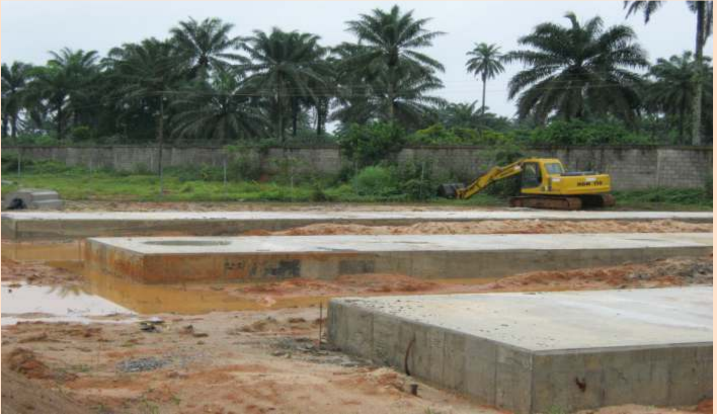
Equipment Foundation for Pig Receiver at Egbema Power Metering Station
