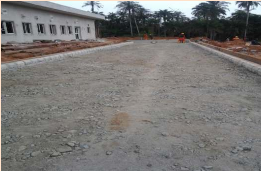
Stonebase Laying At Alaoji Metering Station
