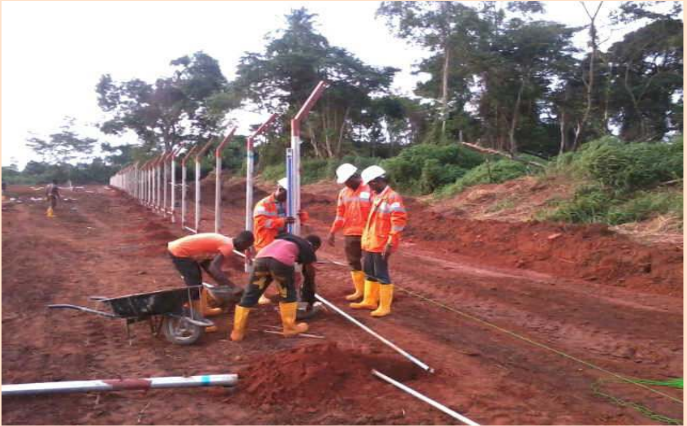
Chainlink F encing
