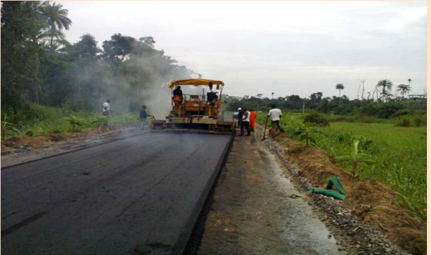
Asphalt Laying At Gbarain Bayelsa State
