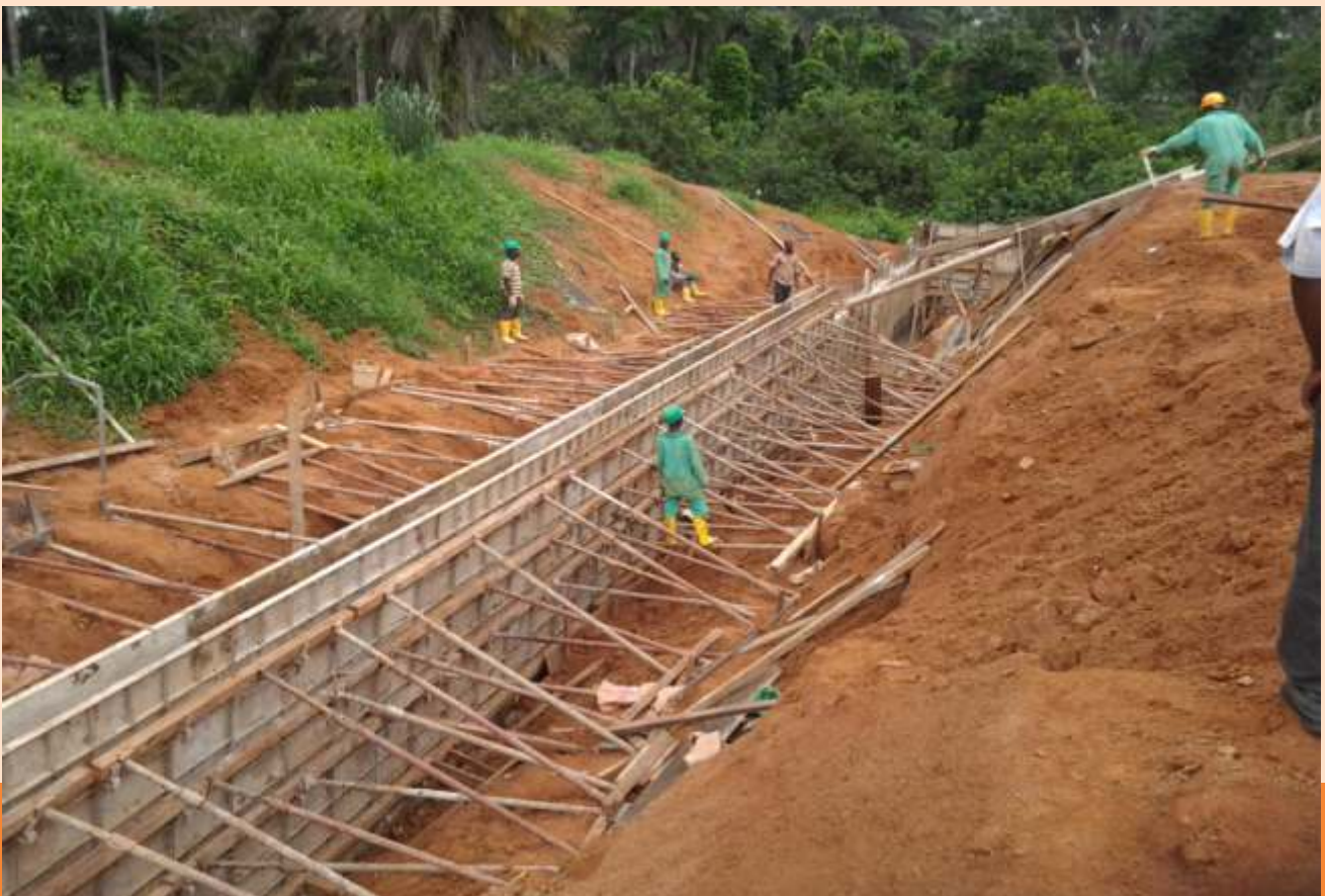
Retaining Wall Construction Against Road Collapse
