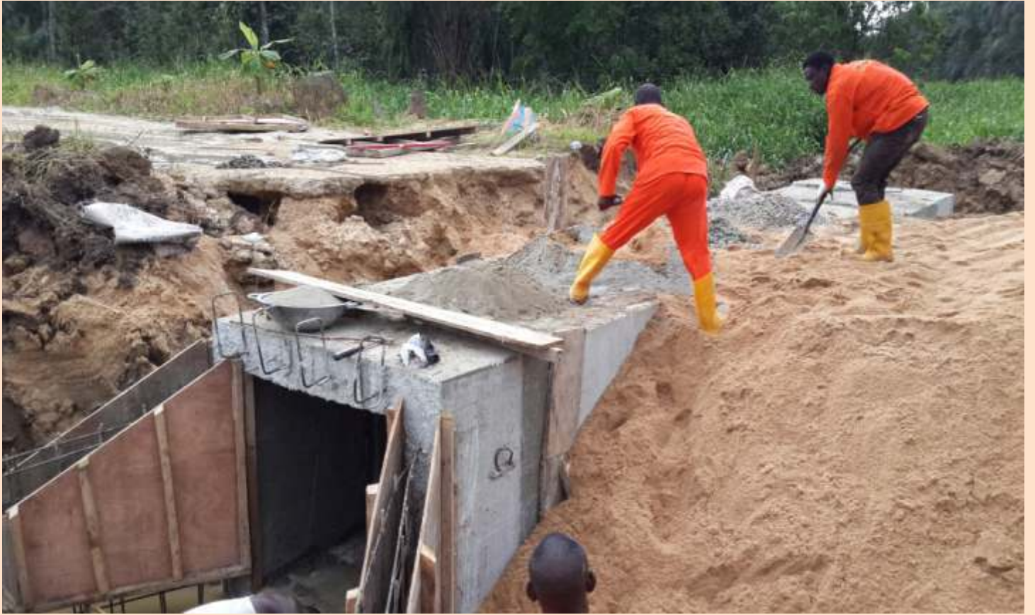
Precast Box Culvert With Wing Wall
