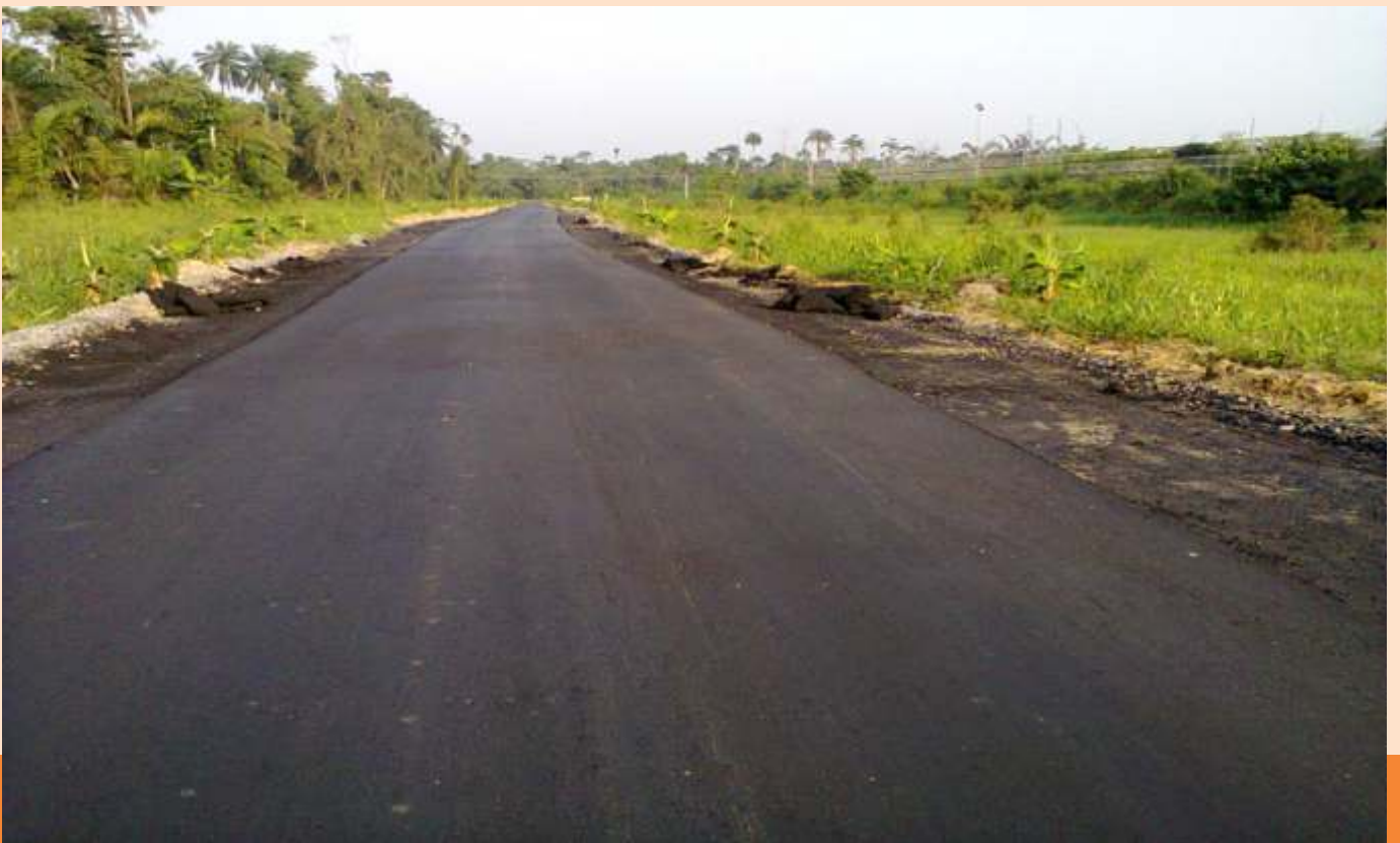
Asphalt Laying At Gbarain Bayelsa State
