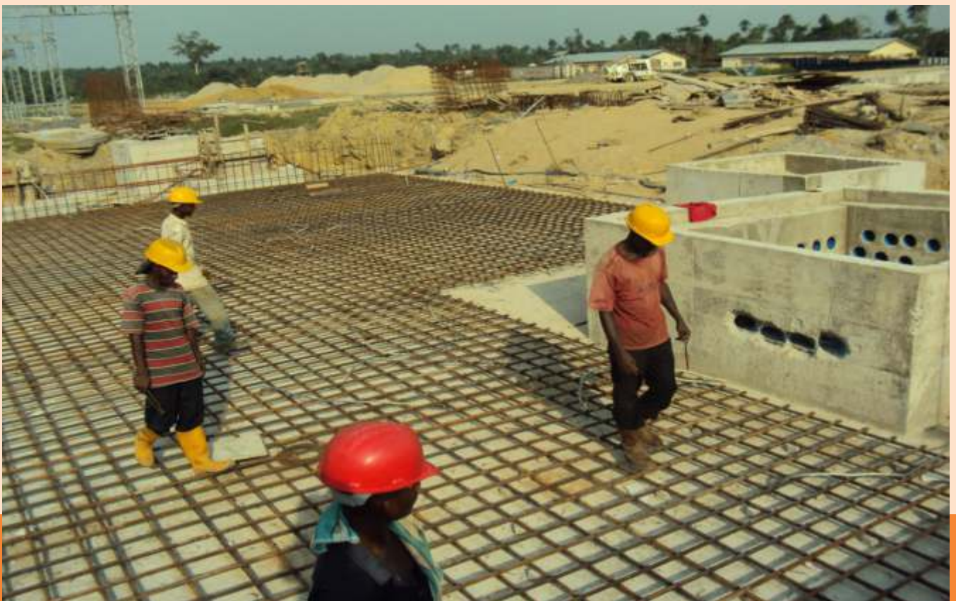
Equipment foundation for Egbeda power metering station installation.
