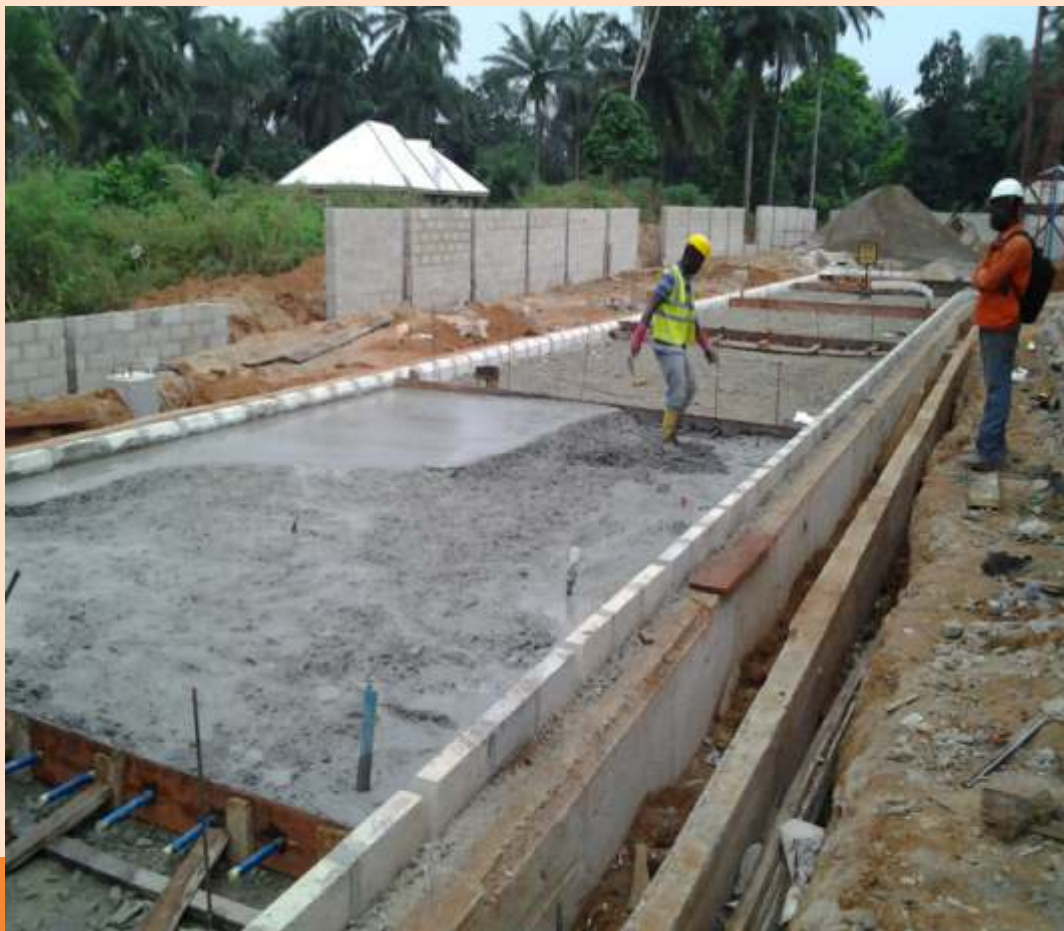
Kerbs Laying On Alaoji Concrete Slab With Dowel Bars
