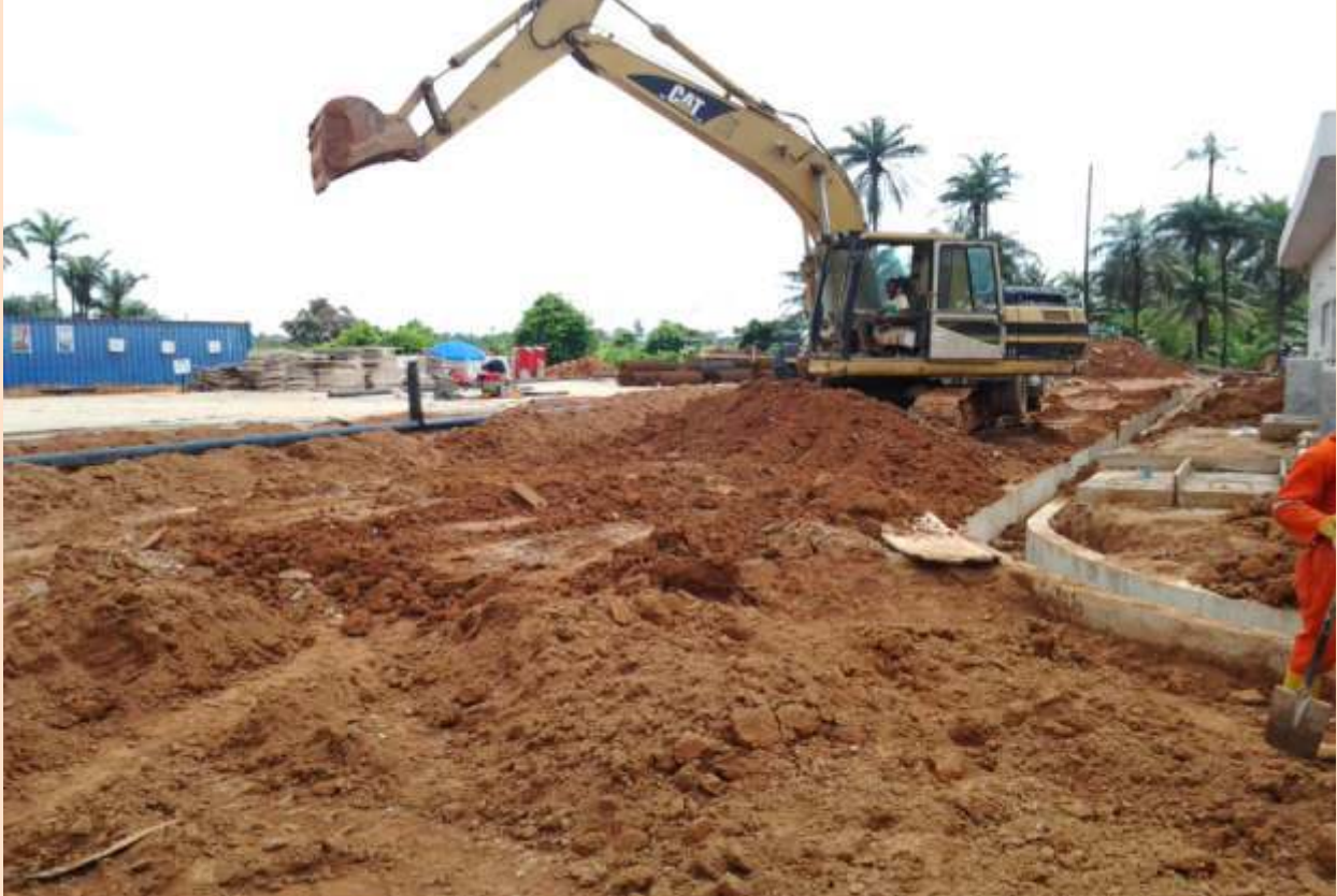
Cutting Down Road To Required Level
