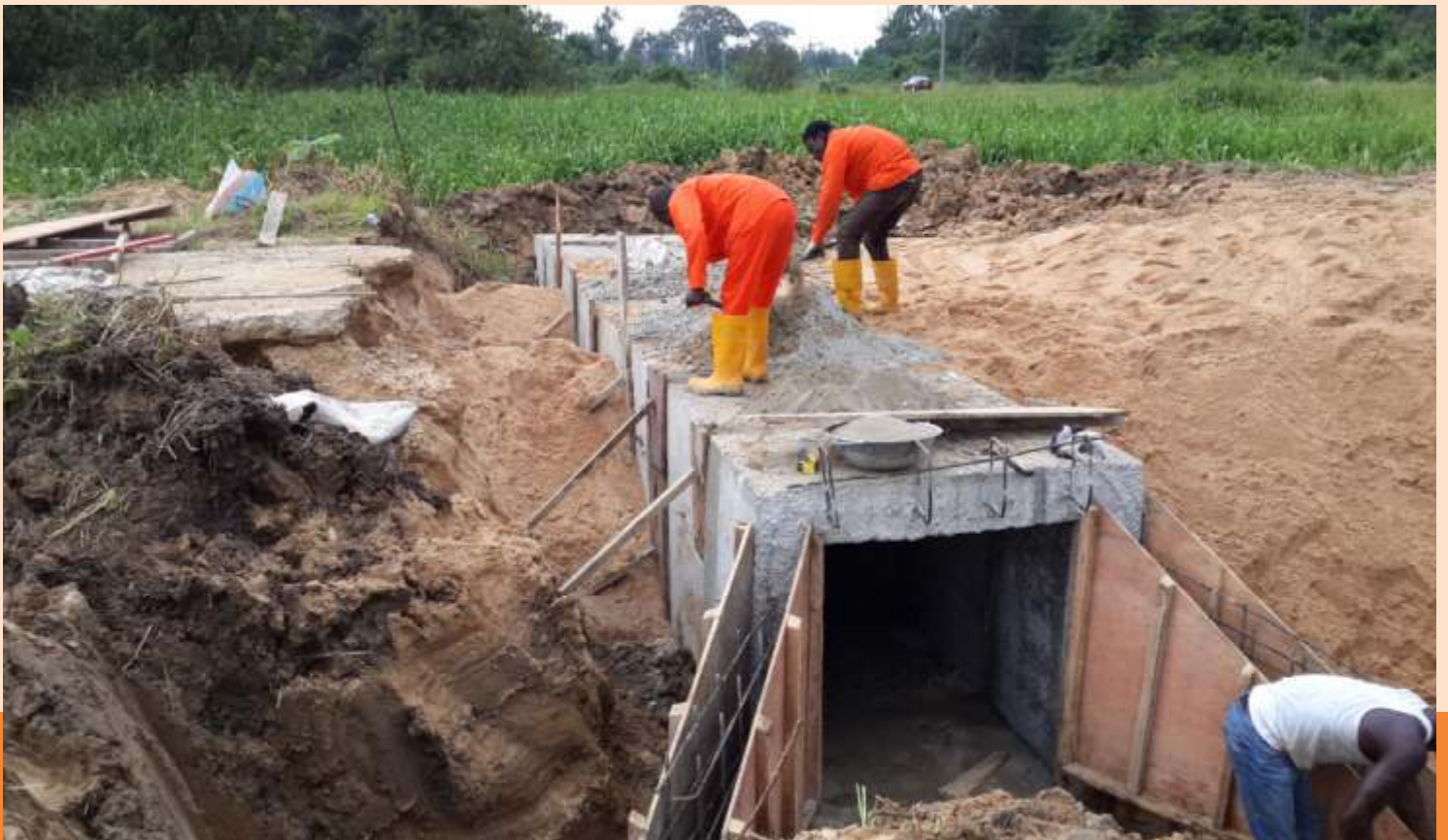
Precast Box Culvert With Wing Wall
