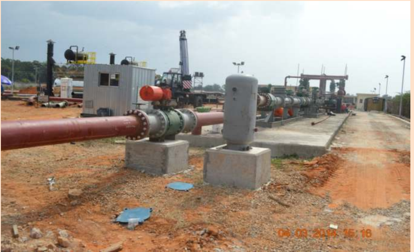
Equipment foundation for Egbeda power metering station installation.
